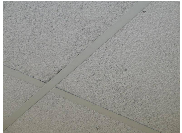
T-bar ceiling showing damaged area
