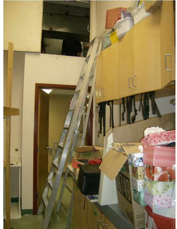
Mechanical Room Access
