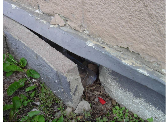
Cementitious cladding at base of 1972 addition
