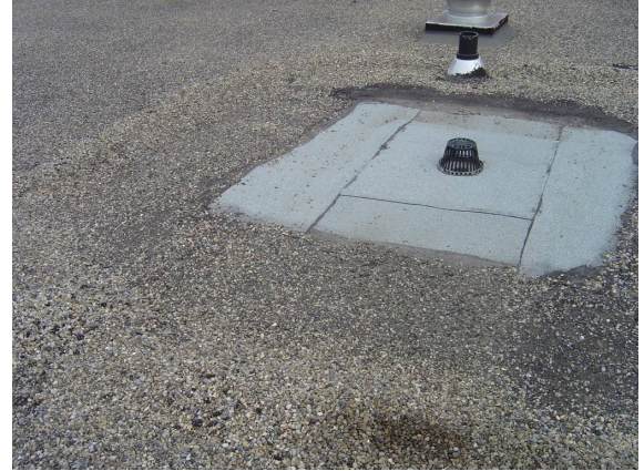
Built-up roof, patched with SBS
