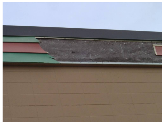
Top of gym wall, east side.
