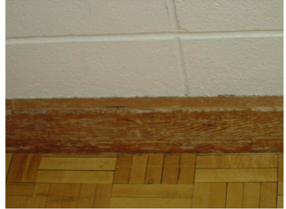
Gymnasium wood wall base.
