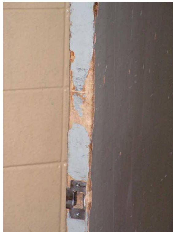
Typical damage to edges of wood doors
