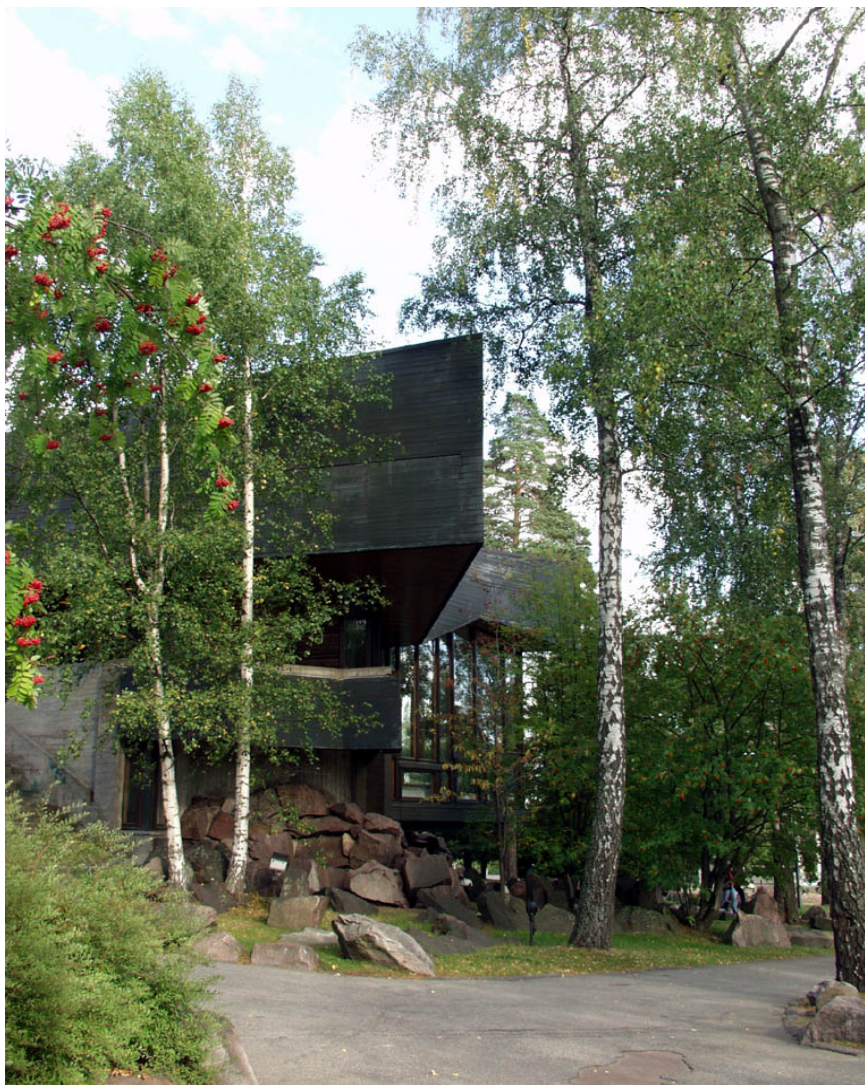
Figure 1.9 Residential building in Helsinki - Although the aesthetics are pleasing and it is blended into the environment; the building is at extreme risk for fire damage and potential loss.
