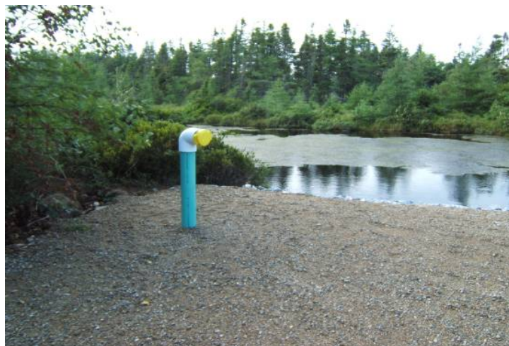
Figure 1.7 Dry Hydrant - An example of a dry hydrant installed on a pond with gravel surface off main road for access. See detailed example in Appendix F
