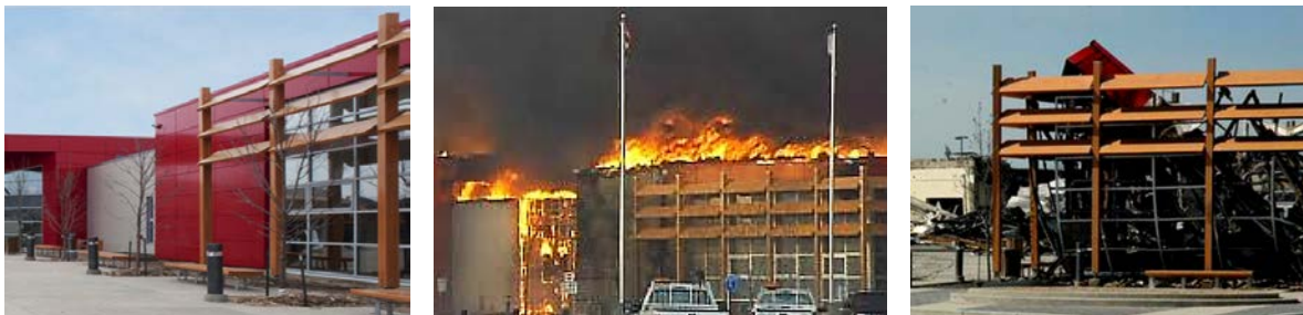
Figure 1.17 Slave Lake Government Centre and Library – Building pre-fire, during fire and post fire
