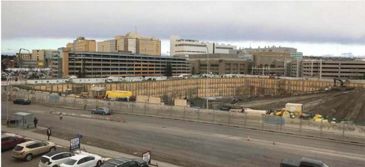
West view of the project site from Foothills Professional Centre, March 26, 2018.
