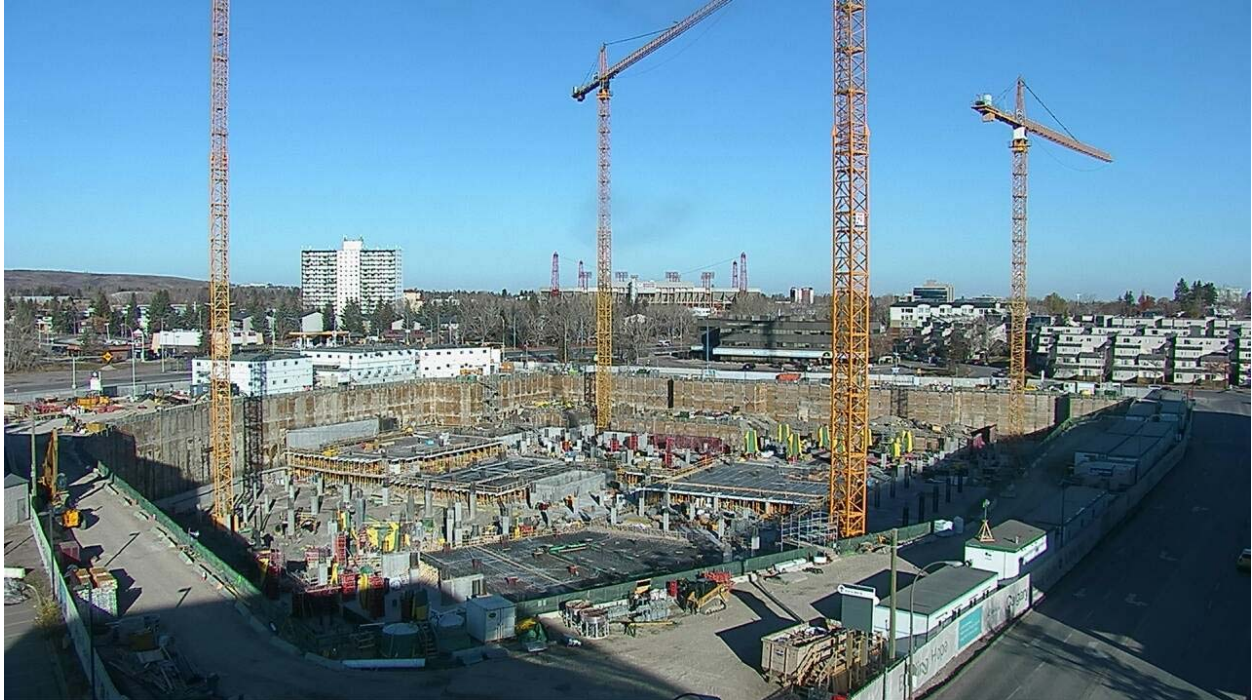
West panoramic view of the construction site, October 21, 2018.
