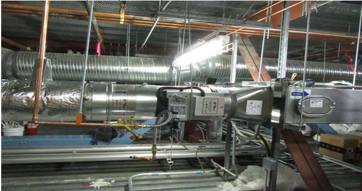
Mechanical and electrical system on the interstitial level at the Stollery Children's Hospital.
