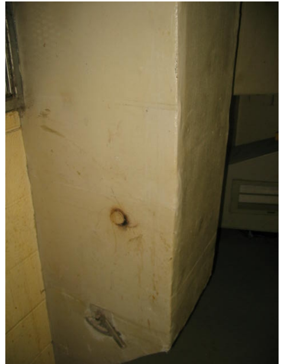
Combustion air duct.
